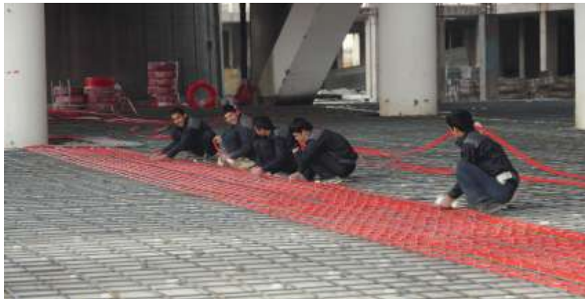
Fig.5: Pipe laying /fastening the cable ties with pipe to the iron mesh
