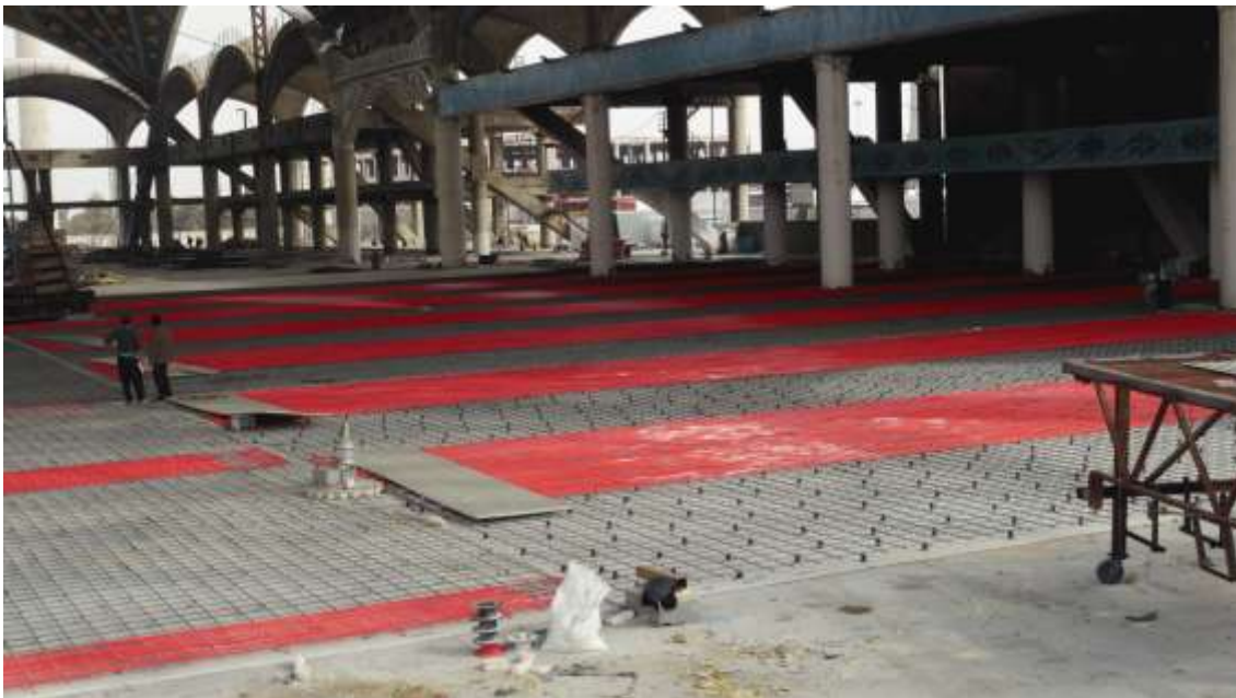
Fig.7: View of the 500 sqm slab with laid pipes
