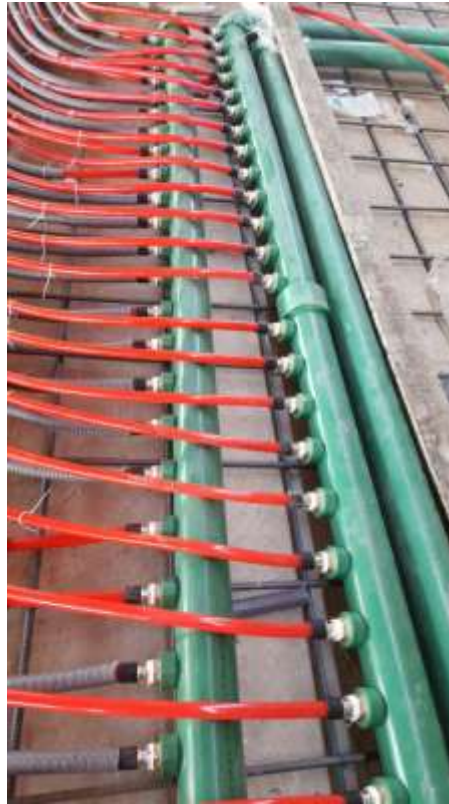
Fig.3: Pipe and manifold connections
