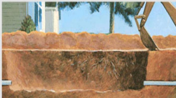
OPEN CUT EXCAVATION
