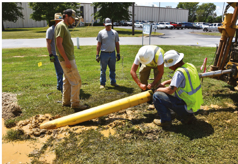
Above: In addition to offshore applications, Evonik's PA12 is used for domestic gas installations
