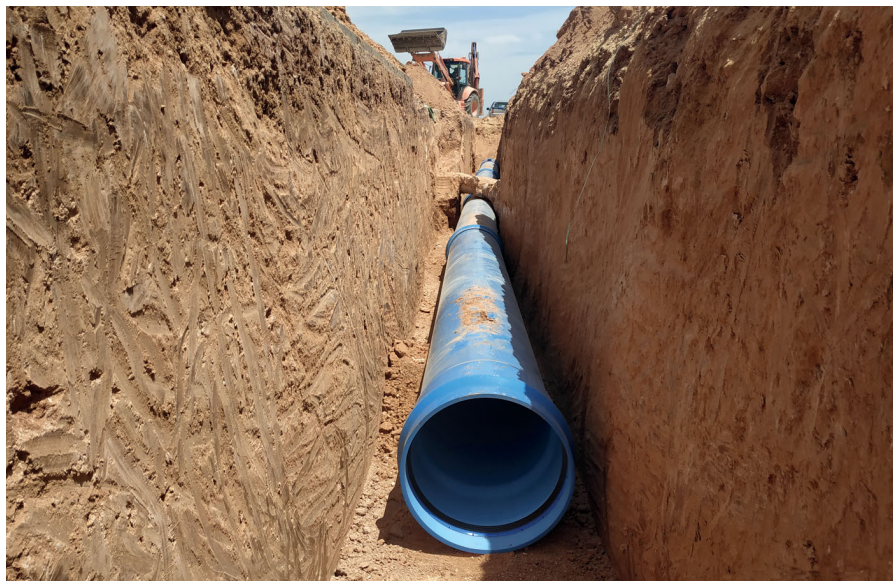
Installation of PVC-O pipes in the modernization project of the irrigable area of the irrigation community of the Tajo-Segura de Librilla transfer
