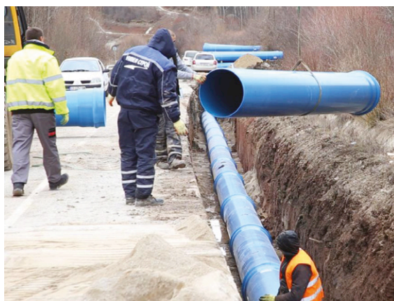
Above and right: Molecor's PVC-O pipe has been used to supply fresh water to Pernik in Bulgaria, after it suffered a severe drought
