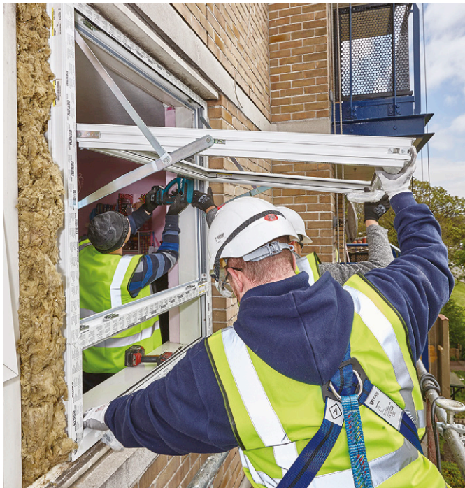
Above: Rehau says that retrofitting PVC window frames helps to reduce carbon emissions
